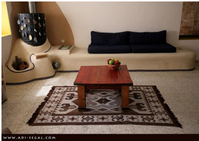
Figure 7: A rocket mass heater with the wood burning part inside the black cylinder at the left, chimney partly visible above and the thermal mass located in the couch. Astonishing performance claims made!
