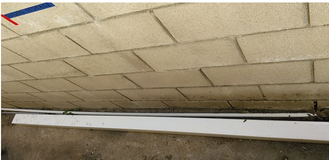
Figure 13: Several lengths of PVC and copper pipe left outside, on the ground, by the back door of my pantry
